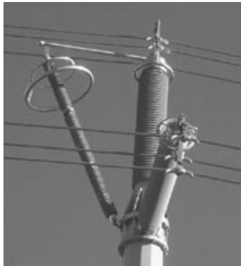
Compact 400 kV tower without overhead shield wire. Insulators protected by TLA in top phase.
